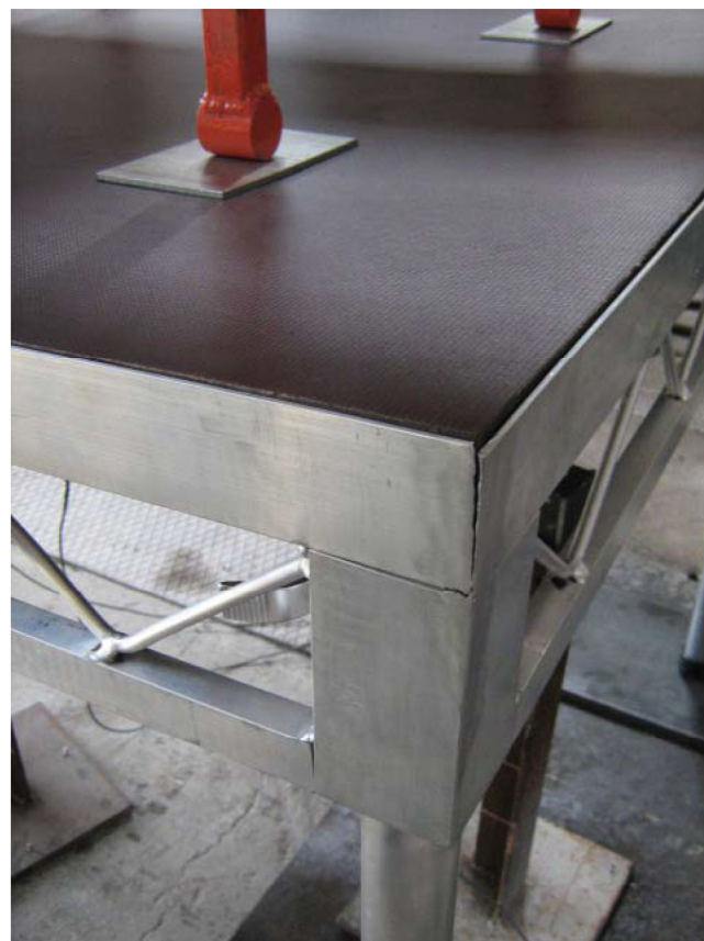
Figure 13 Failure of Welds of Global Truss Performer Stage
