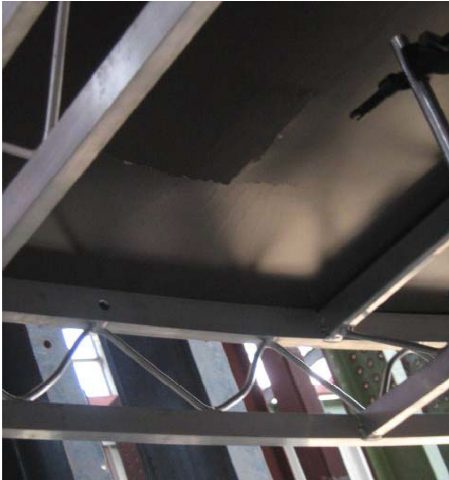
Figure 14 Failure of Timber Platform of Global Truss Performer Stage
